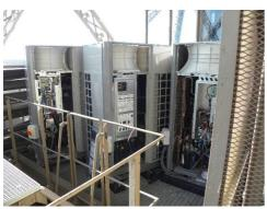
Variable refrigerant flow (VRF) system composed of three modules with a 56 Horse Power capacity installed outdoors and coupled with a heat recovery
